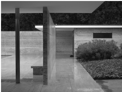
Figure 5. German Pavilion, Barcelona, 1928–1929, reconstruction 1983–1986, L. Mies van der Rohe, view of the service annex in the background (courtesy of Christian Gänshirt, 2012, via Wikimedia Commons).
